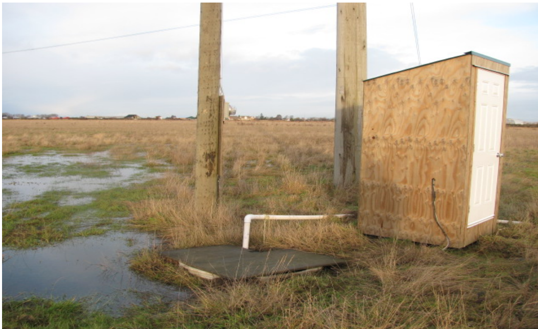
Picture 5 - Roberts Bank – Drainage tile installation and pump house – O&M
