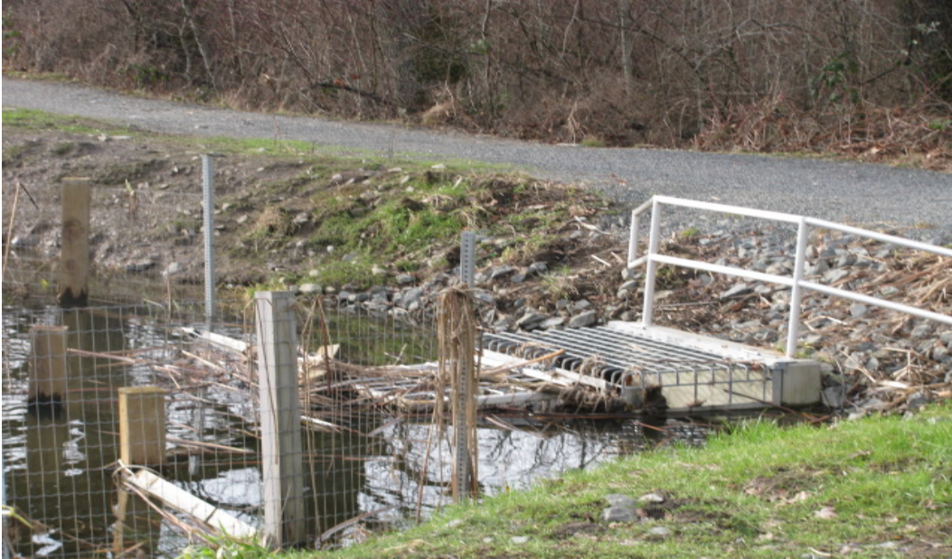
Picture 7 – Buttertubs - Rebuild
