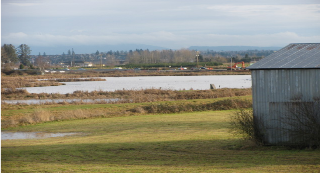
Picture 1 – Serpentine dykes and area that require mowing - O&M
