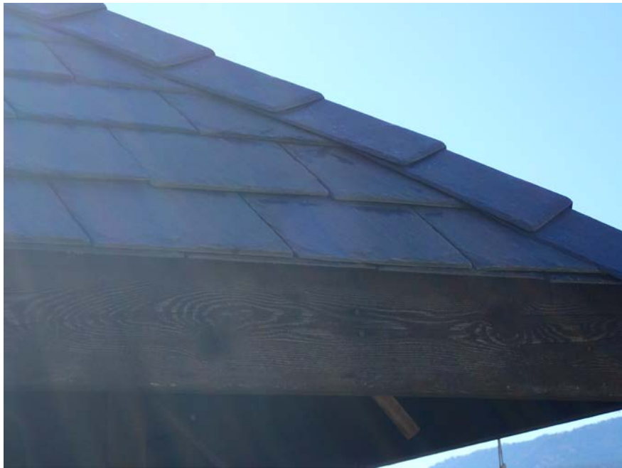
Figure 17. View of kiosk roof showing shingles and cap on hip.
