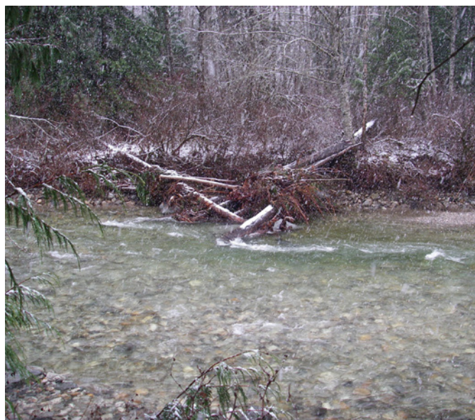
Large woody debris structures, Silverhope Creek
