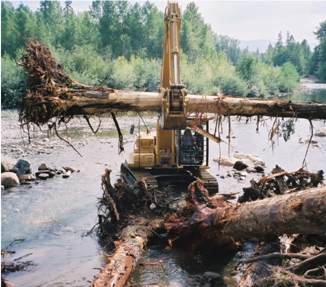
Placing large woody debris, Englishman River
