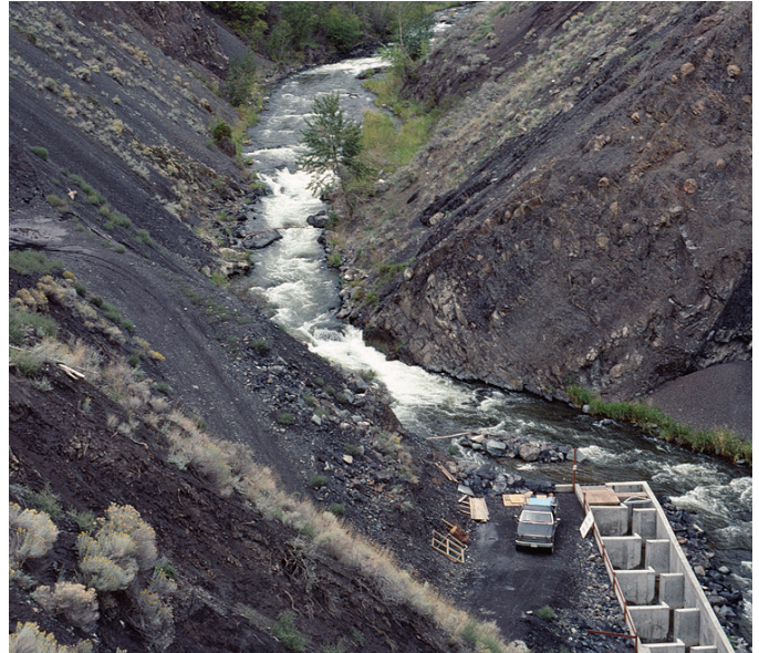
Bonaparte fishway construction, Bonaparte River
