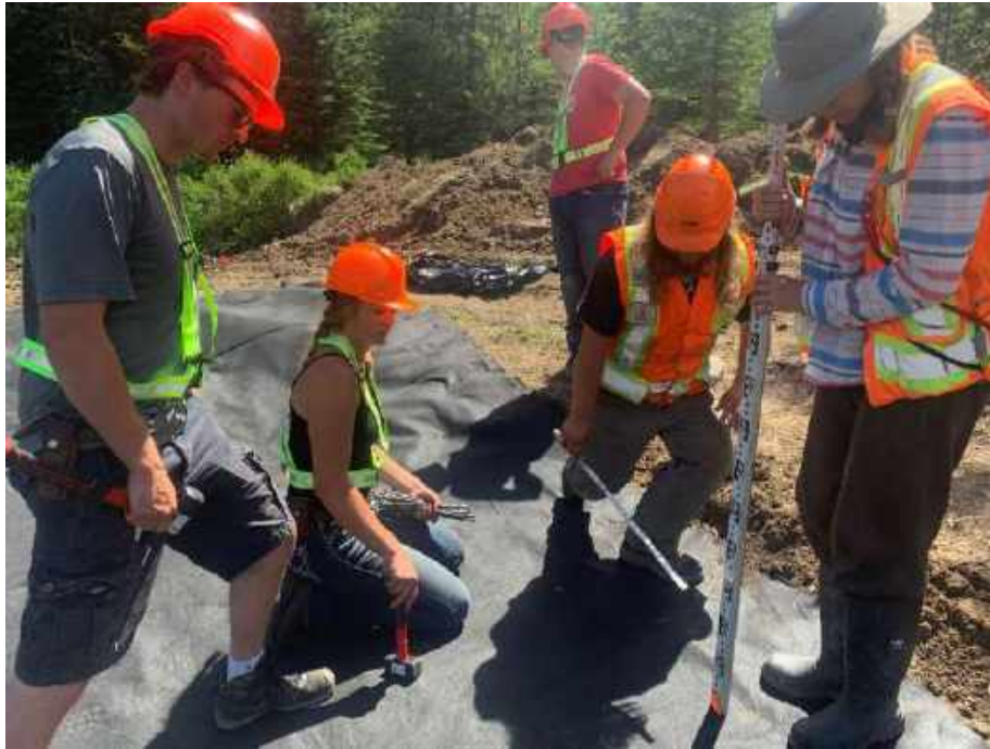
Figure 17: NTBC Crew helping lay a fish-grade pond liner for the Big Ranch wetland enhancement project.
