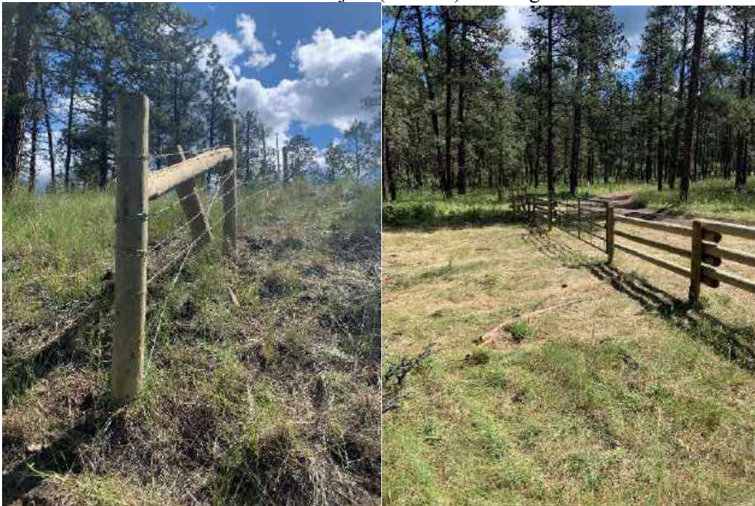
Figure 15&16: New wildlife friendly fence constructed at Wasa Slough, through T4W funding.
