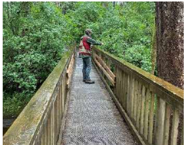
Willow Creek Bridge vertical slats replaced with horizontal rails
