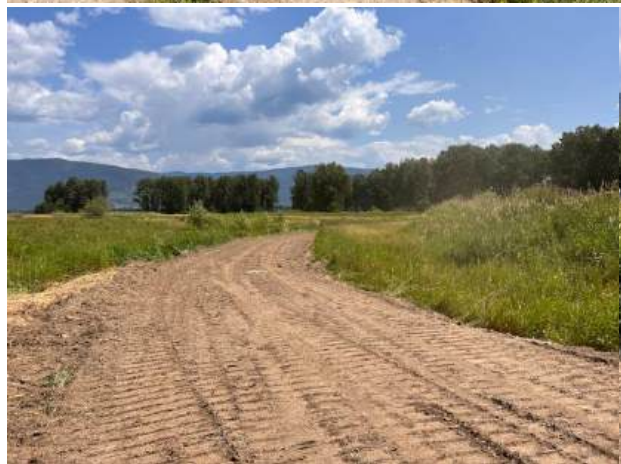
Figures 16-19: At Creston Valley WMA, eroded dike access to the Leach Lake wetland unit (top left) on 26 June 2023. Temporary dike access to Leach Lake being built around the eroded dike on 6 July 2023 (top right) and completed access (bottom left and right) on 6 July 2023.
