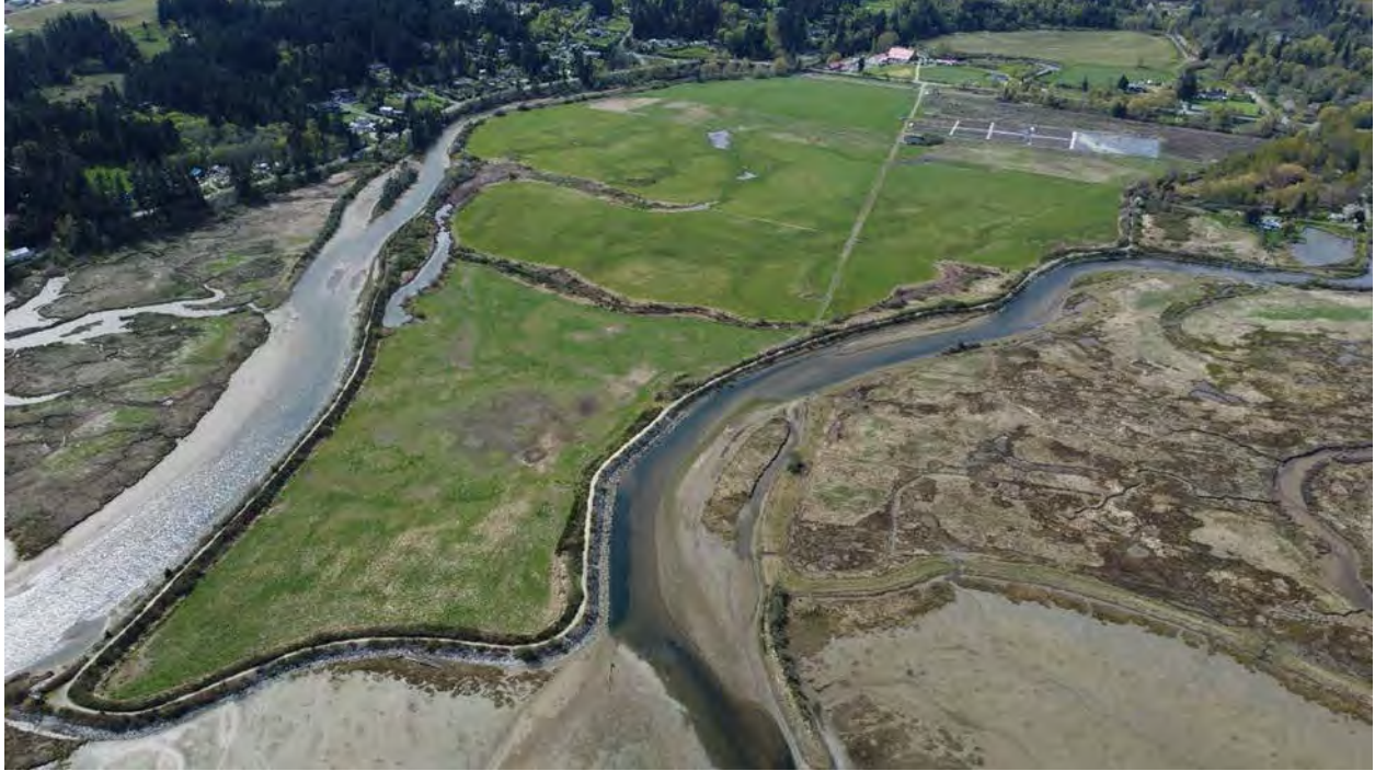
Figure 6 Cowichan Estuary restoration site with perimeter dike and isolated fields within
