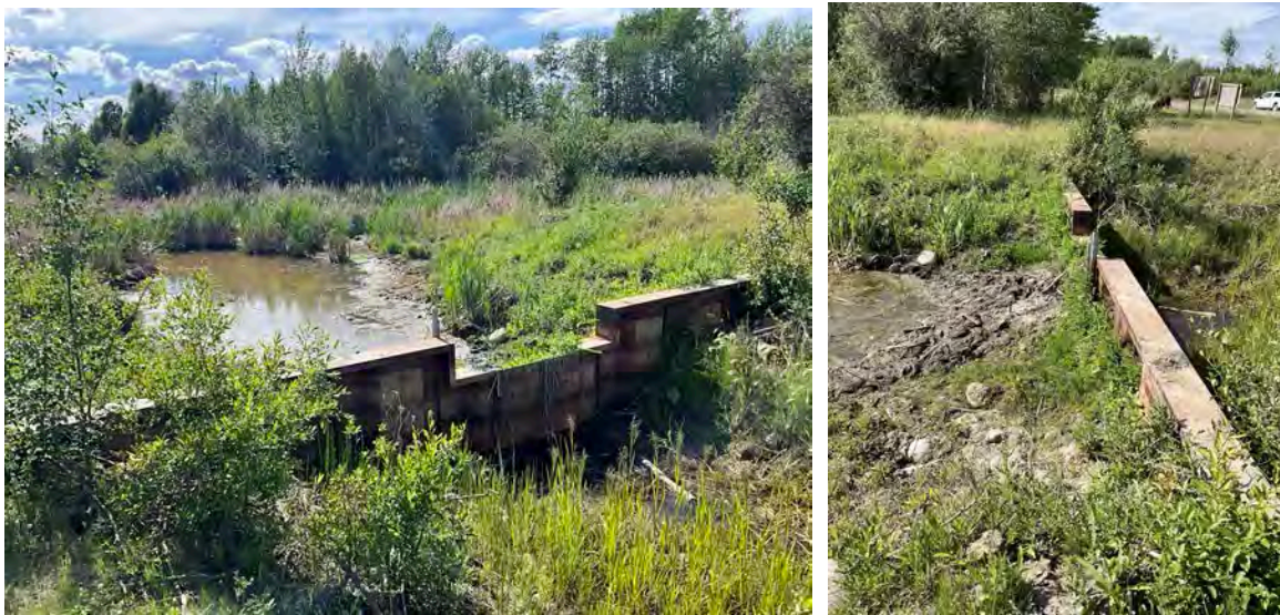
Water weirs at Boundary Lake (left) and Worth Marsh (right). Note beaver debris for removal and overall low water levels in 2025.
