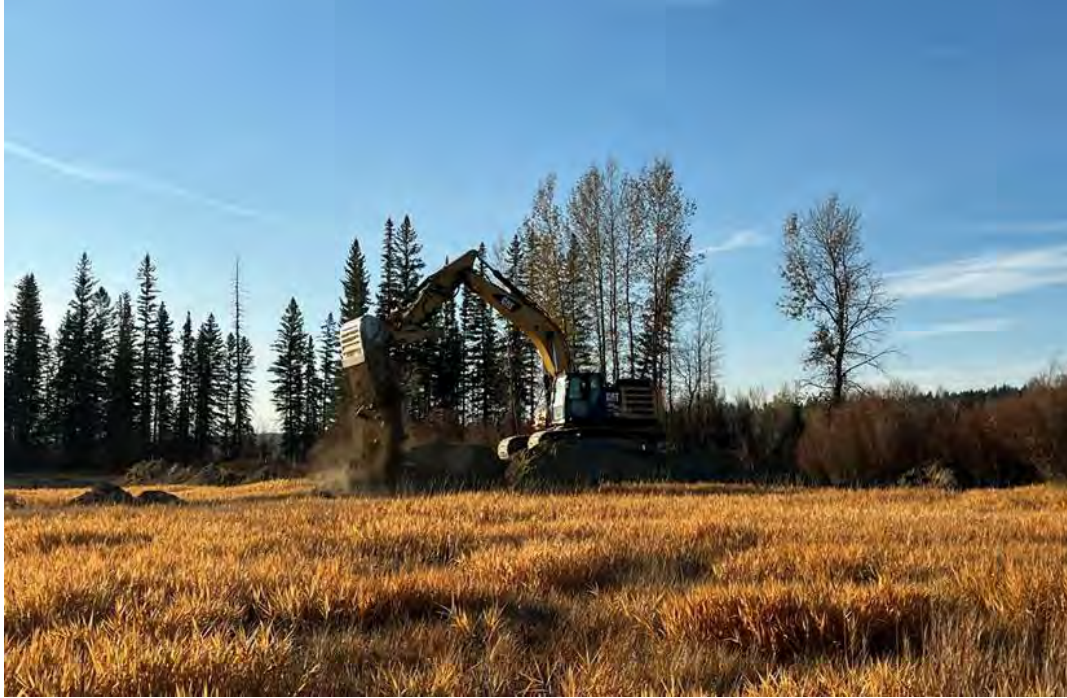
Figure 11. Heavy equipment mobilized to Bummers Flats - North in October 2025 to undertake the first phase of wetland basin excavation, removal of old water control infrastructure, and to implement breaches in dikes, all with the purpose of restoring a more natural flood cycle. Ducks Unlimited Canada Photo.
