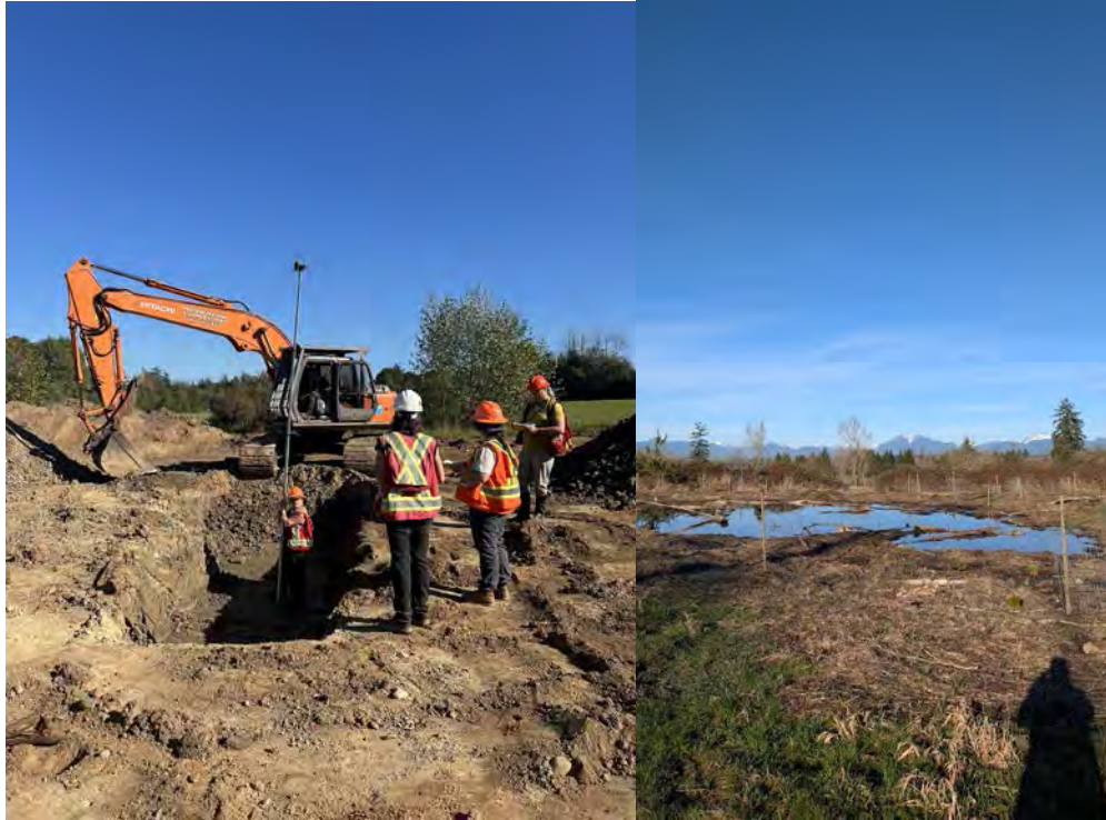
Wetland construction at Forslund-Watson Conservation Area in partnership with BCIT (Photo on left: during construction; right: Photo on right: three months post-construction).
