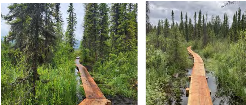
Cranberry Marsh WMA wooden plankway installation
