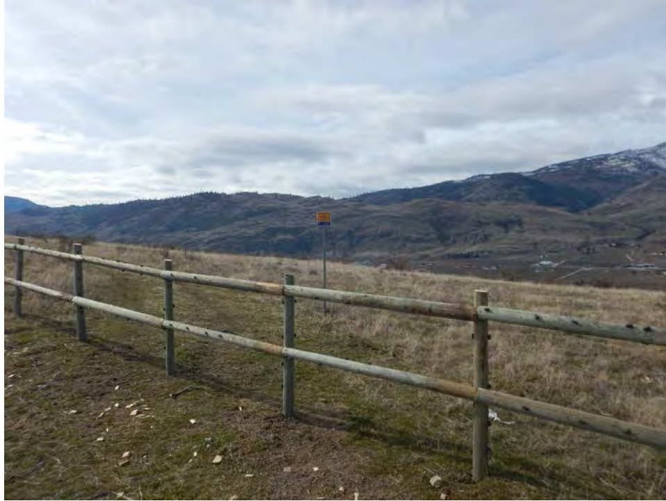
Figure 16. New fence and sign installed in 2026 blocking the unauthorized access at the SOWMA parcel near the Oliver Landfill.
