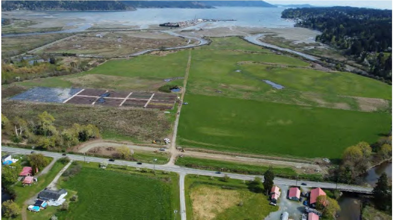
Figure 6 Cowichan Estuary with Phase 1 construction in foreground underway
