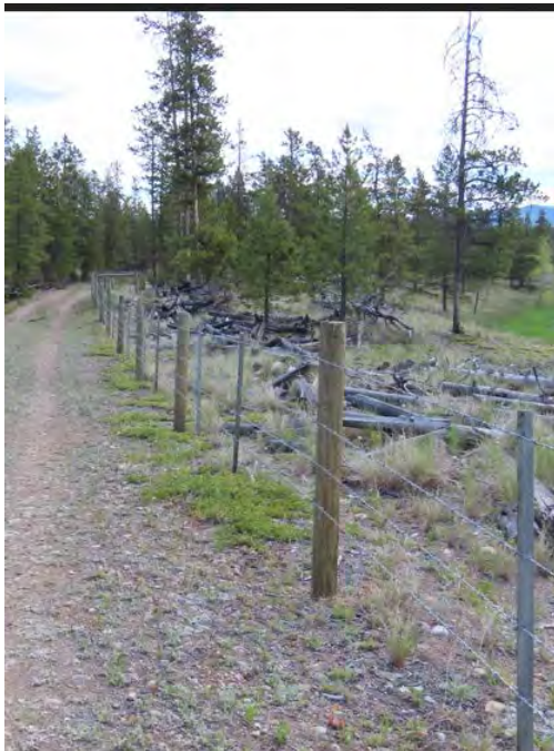
Chilanko Marsh WMA livestock exclusion fencing
