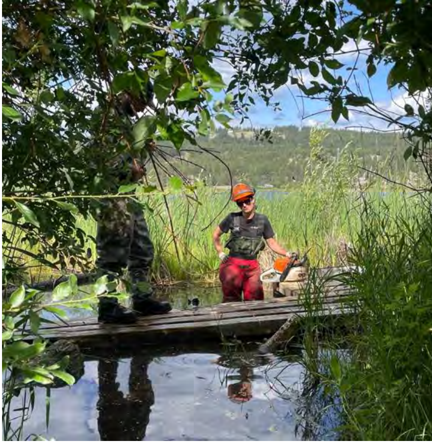
Figure 9. Removal of the dilapidated dock at Elizabeth Lake posed some logistical challenges that were overcome by a certified chainsaw operator from BC Wildfire Service who volunteered her time.
