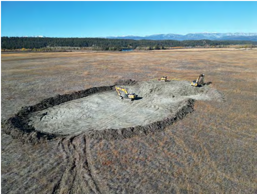
Figure 12. Basins were excavated to support a longer hydroperiod and contribute to a greater diversity of habitats. Photo by Kerr Wood Leidal Associates Ltd.
